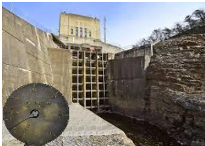
The gage, gate & creek.
